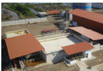
Stasiun Waste Water Treatment Plan
