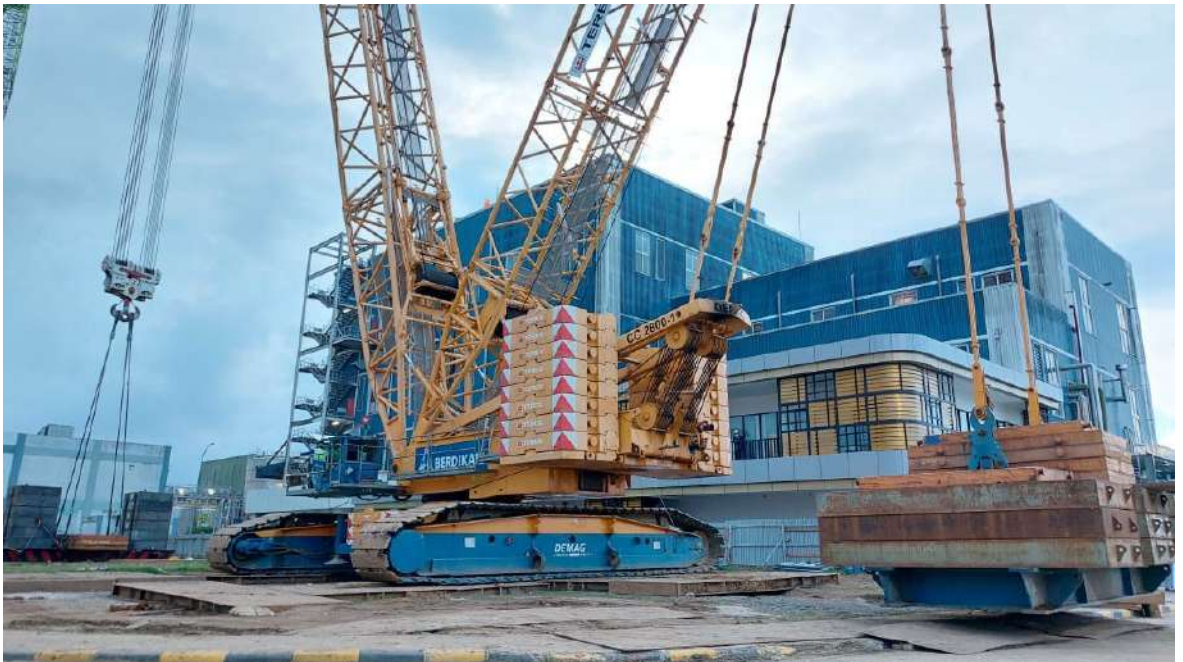
Gambar 4. Heavy Lift Crawler Crane
